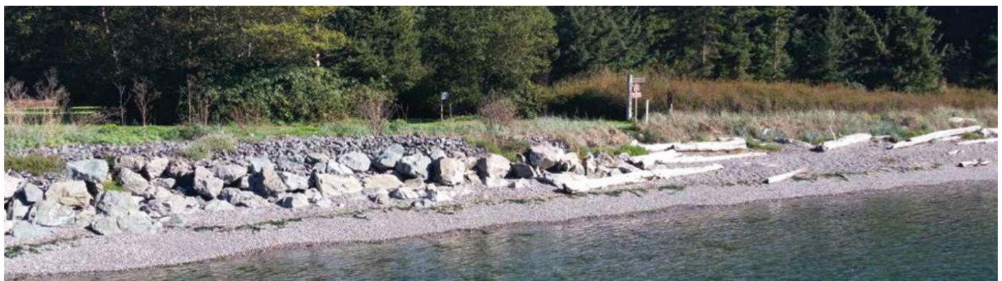
Figure 8. Hard protection measures (left) and soft protection (right) on neighboring Washington beachfront properties.
