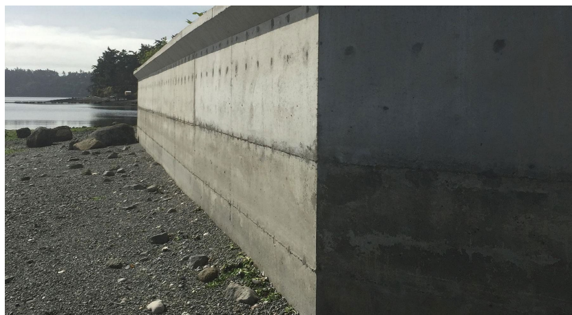
Figure 13. Photo of a bulkhead along Washington’s coast.
