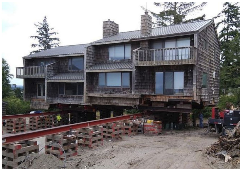
Figure 24. Photo of a building being moved back from the coastline performed by DB Davis Structural Moving & Raising Company.
